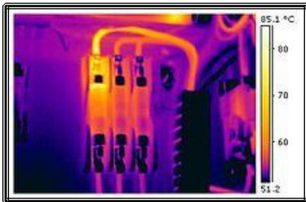
This thermogram shows excessive heating on a terminal in an industrial electrical fuse block. from <https://en.wikipedia.org/wiki/Thermography>
