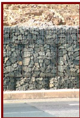
Physical barriers of many sorts are used, from rocks and trees to cages made from materials as diverse as wickerwork, concrete and metal. Such 'cages' are known as 'gabions', and come in many forms. Retaining walls, flood walls and dams are all built by civil engineers to prevent erosion by water and other natural forces.
